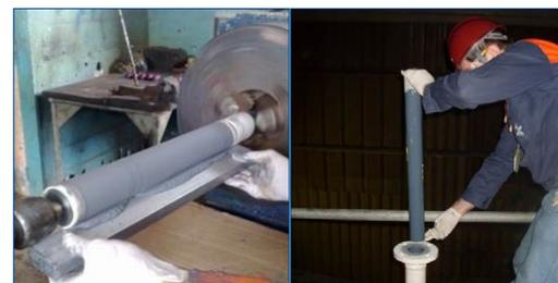
In order to protect small bore nozzles, a conventional coating would not be sufficient due to the risk of pinholes or holidays when coating a narrow nozzle. This issue is rectified by introducing prefabricated nozzles made from Belzona composites that do not corrode. The inserts and the nozzle are wetted out with a Belzona coating grade material, before being installed and bonded together to ensure corrosion protection.
