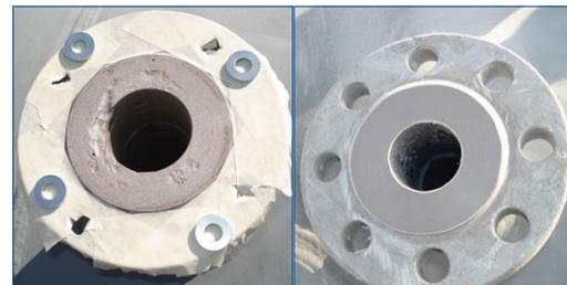
Flange face corrosion is a common problem affecting pressure vessels, where the face must be isolated to prevent oxidation. Belzona composite materials do not corrode and bond strongly to the flange face, where prefabricated formers are used to shape specified Belzona material on the flange face.
